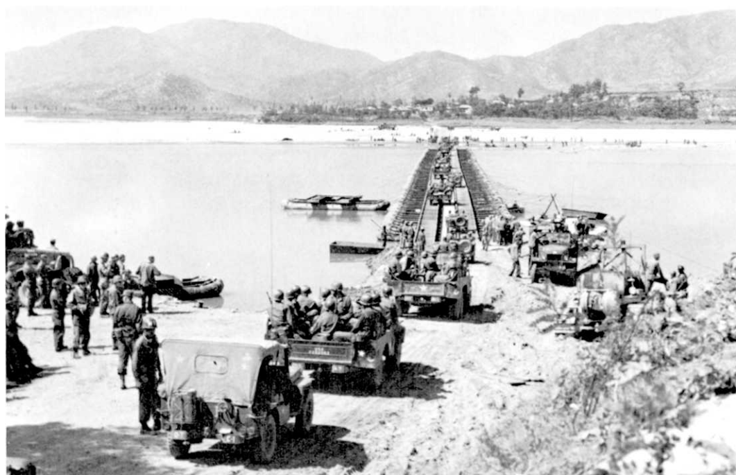
PONTON TREADWAY BRIDGE across the Naktong, built in thirty-six hours.
