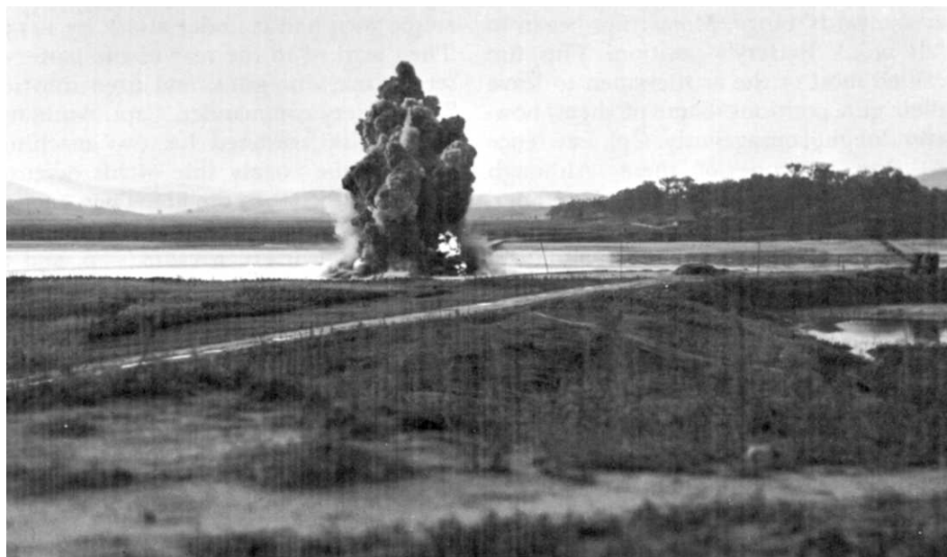
KUM RIVER BRIDGE EXPLOSION
