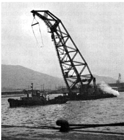
60-TON CRANE AT PUSAN
